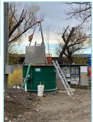
Kalavista Lift Station upgrades – extension to the existing wet well
