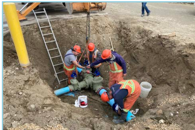
District crews installing a watermain gate valve for a fire hydrant on Westkal Road
