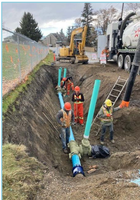
District crews installing a new water service and fire hydrant on Kidston Road
