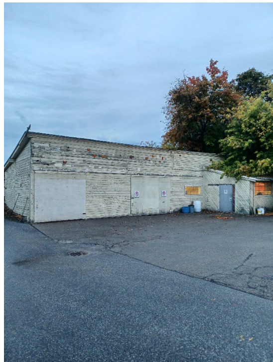
Old storage building
