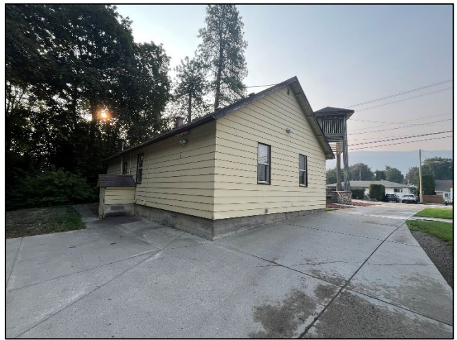
MAIN BUILDING REAR CORNER VIEW
