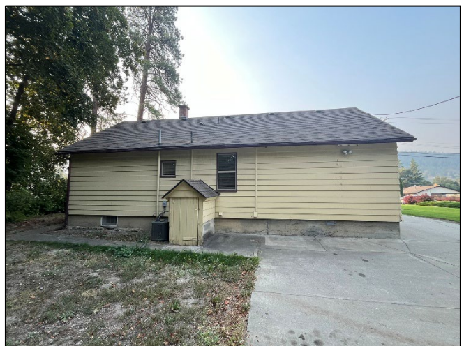
MAIN BUILDING REAR VIEW
