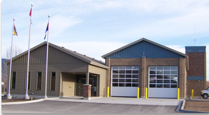
Lavington Fire Hall on School Road
