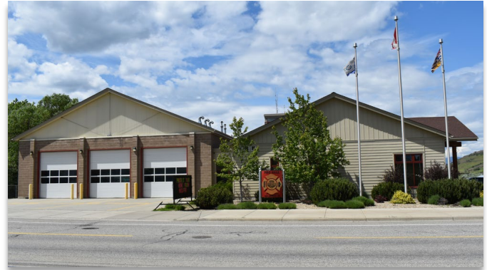
Coldstream Fire Hall on Aberdeen Road
